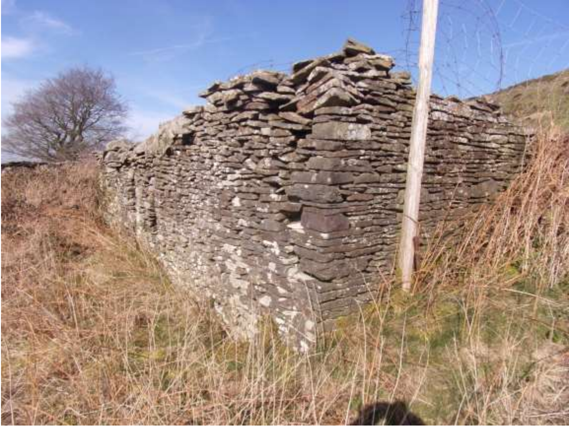
Figure 7 Remains of south-east gable wall. (RJS)
