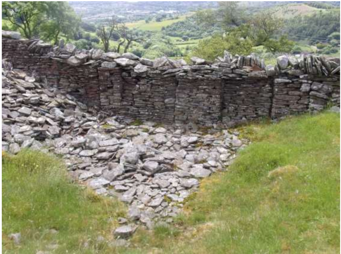
Figure 2 the blocked up door way and windows from inside (RJS)
