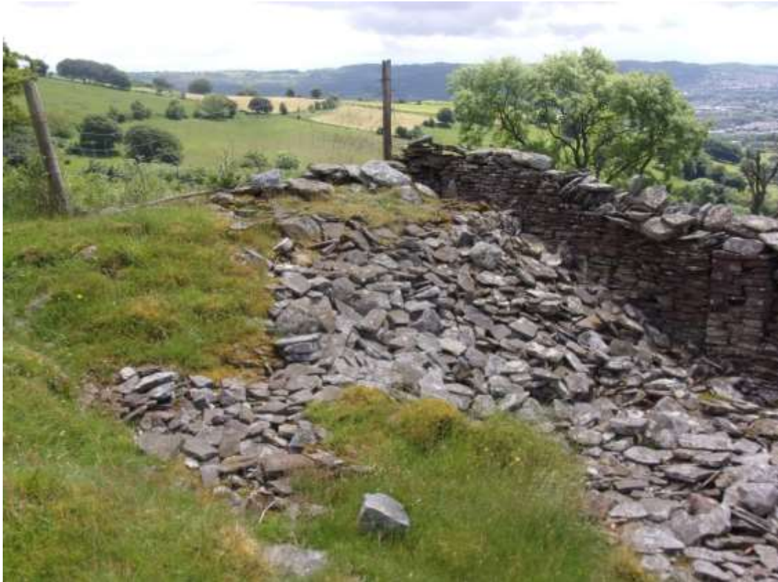
Figure 3 fallen south-easterly gable wall. Possible location of fireplace and chimney (RJS)
